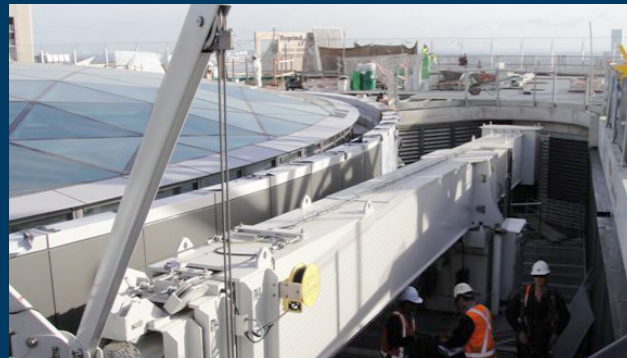
1 Bligh St, Sydney – parked in a pit and then erect
